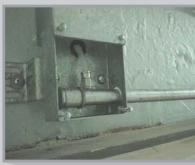
**Hidden sampling**A tiny Xtralis VESDA sampling capillary is hidden behind a light fitting, invisible to unsuspecting occupants.
